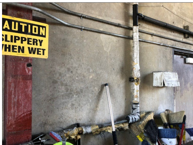
Fiberglass Pipe Wrap
