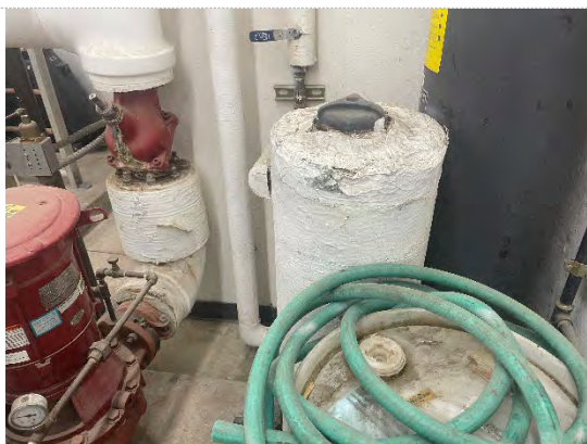
Fiberglass Pipe Wrap – 2"
