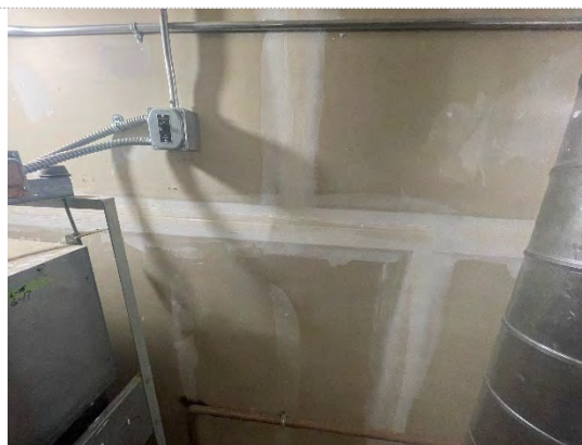
Unfinished Drywall with Tape and Joint
