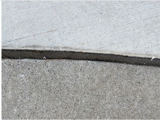
Fibrous Expansion Joint
