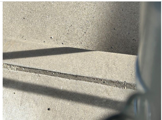
Fibrous Expansion Joint
