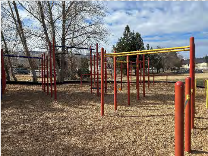
Burnt Orange & Dusty Yellow Paints on Metal Play Structure
