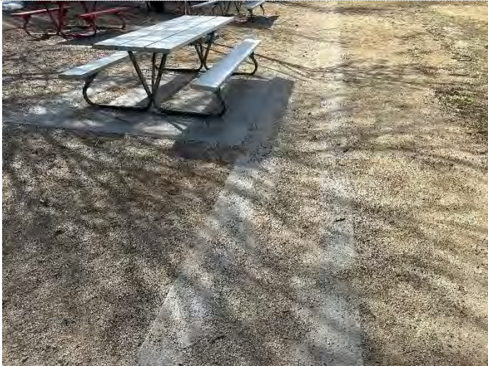
Concrete Valley Gutters
