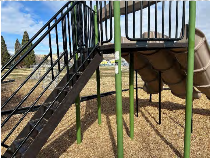
Dark Brown Vinyl Coating Green & Black Paints on Metal Play Structure
