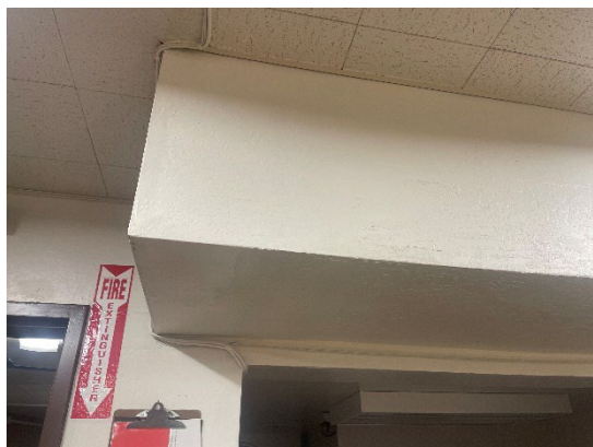
Drywall – Orange Peel Texture w/ T&J and White Paint on Drywall Wall
