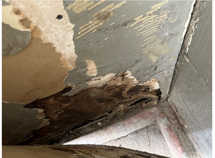
Damage & Mold Growth on Drywall Wall
