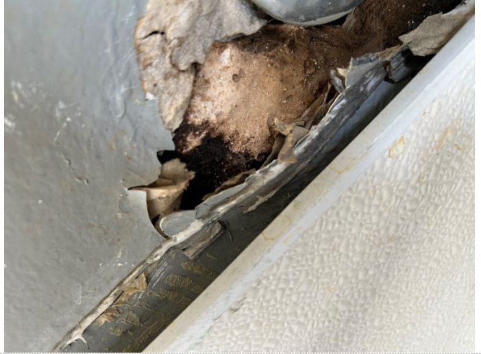
Damage & Mold Growth on Drywall Wall
