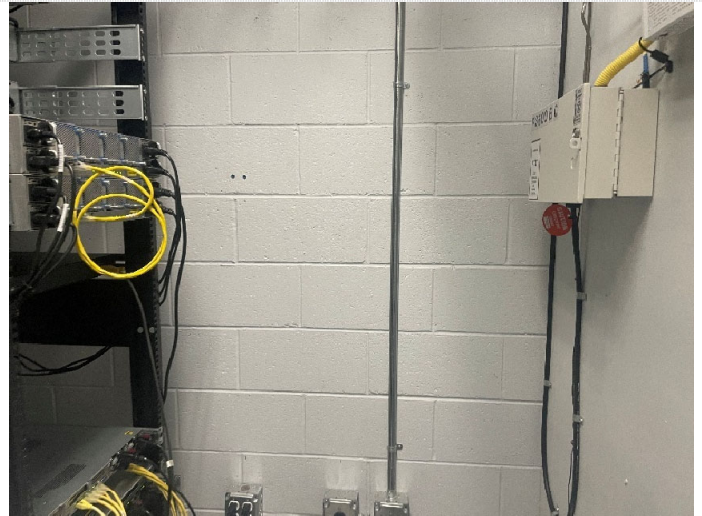
Light Grey Paint on CMU Wall
