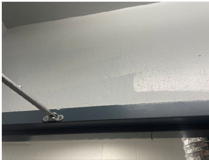
Grey Paint on Metal Door Frame Light Grey Paint on Drywall Wall
