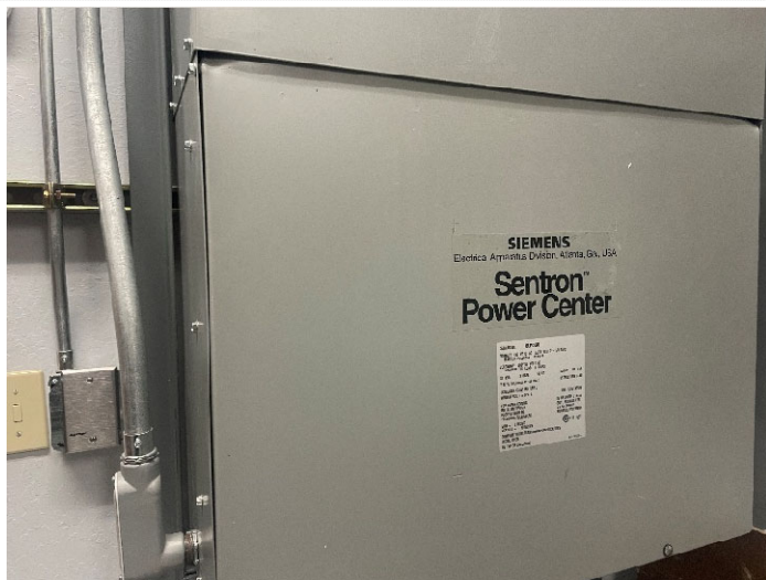
Grey Paint on Metal Electrical Box
