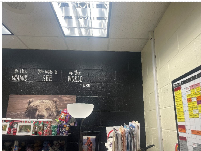
Black Paint on CMU Wall
