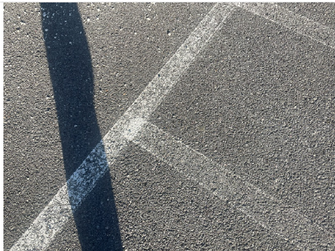
White Paint on Asphalt Parking Lot
