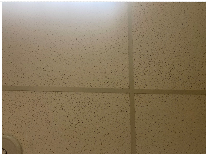
White Paint on False Ceiling Panel 4'x6' False Ceiling Panel – White
