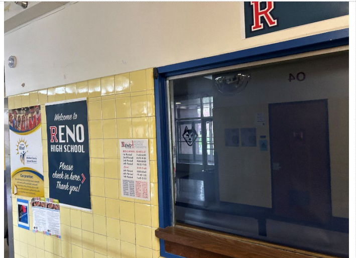
Blue Paint on Metal Windowframe
