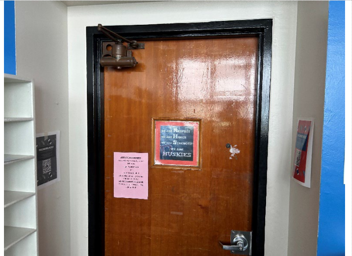
Black Paint on Metal Doorframe Clear Varnish on Wood Door
