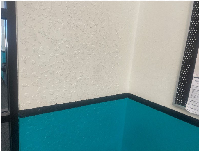
Black Paint on Drywall Wall White Paint on Drywall Wall
