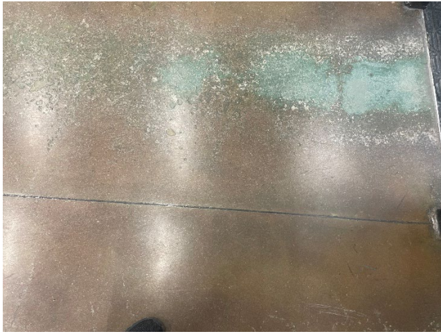
Tan Coating on Concrete Floor
