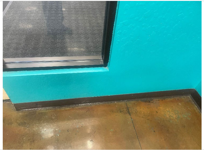
Teal Paint on Drywall Wall 4" Baseboard and Mastic – Black Black Paint on Metal Door/Window Frame
