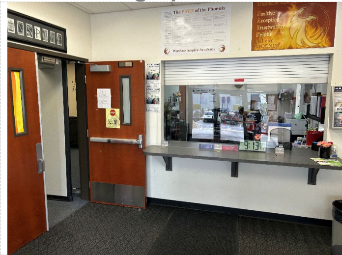
Drywall – Knockdown Texture White Paint on Drywall Wall
