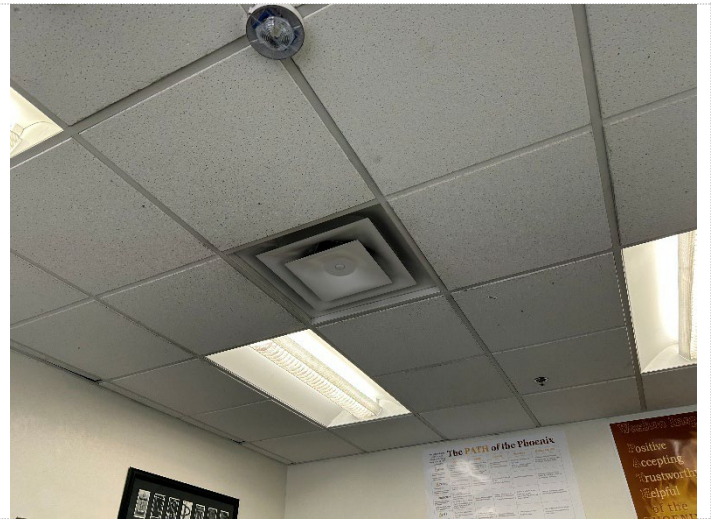
2'x4' False Ceiling Panel – Pinhole Fissure White Paint on False Ceiling Panel
