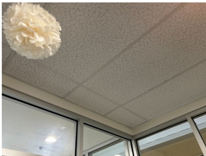
2'x4' False Ceiling Panel – Pinhole Fissure White Paint on False Ceiling Panels
