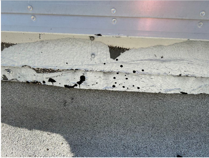
Silver Paint & Mastic
