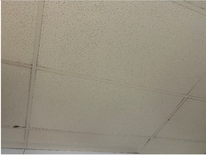
Off-White Paint on Metal T-Grid False Ceiling Panel
