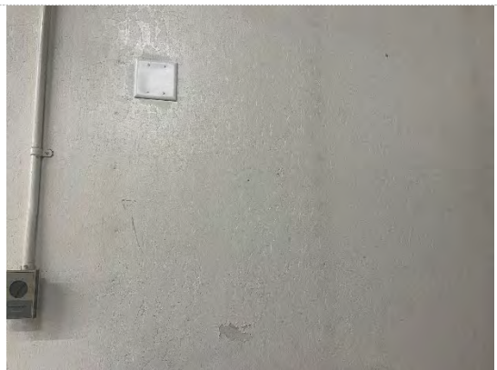
White Paint on Drywall Wall
