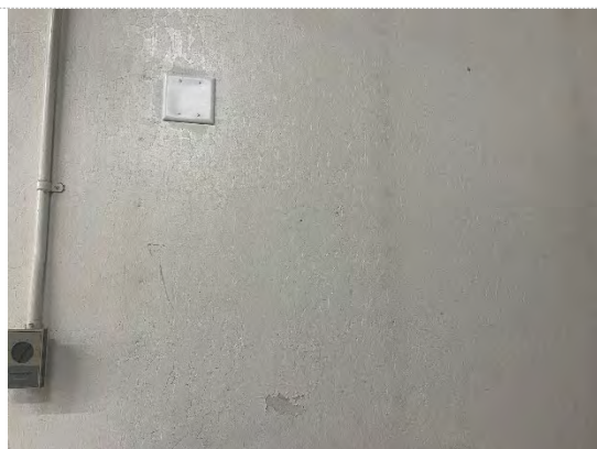
Drywall – Heavy Knock Down Texture – With Tape & Joint
