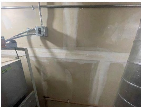
Unfinished Drywall with Tape and Joint
