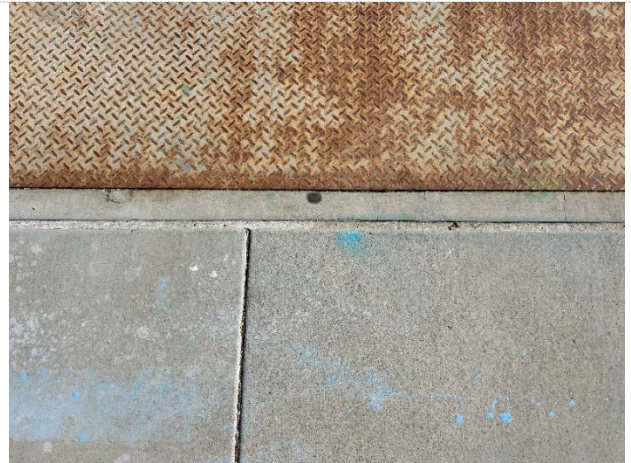
Concrete Expansion Joint
