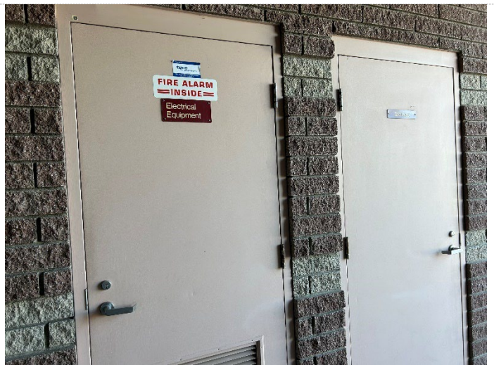
Salmon paint on metal door
