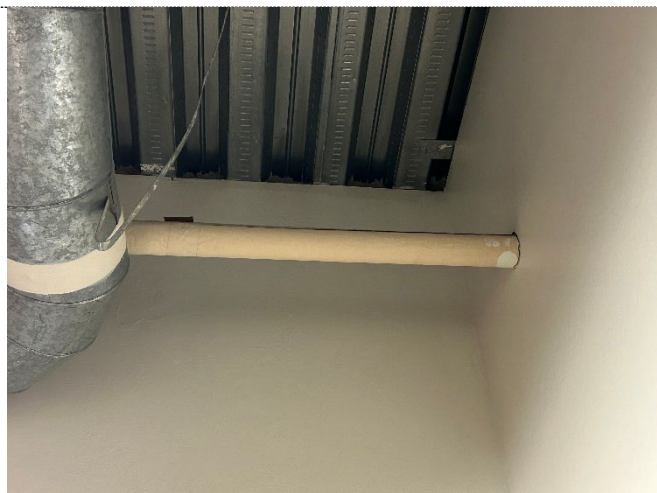
Fiberglass Pipe Wrap
