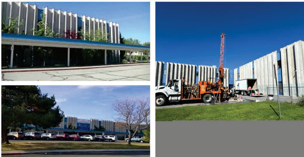
Figure 2: Representative photographs of site conditions
