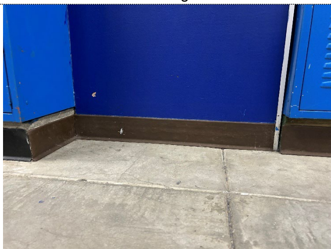
Baseboard & Mastic – 4” Brown
