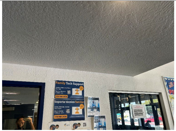
Drywall – Heavy Knockdown Texture
