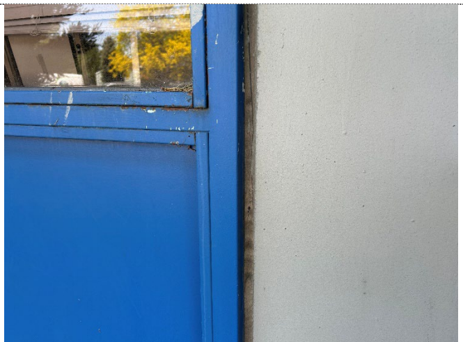
Wall Expansion Joint
