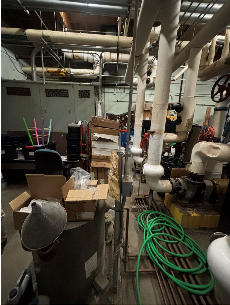
Access from front of domestic water boilers to entry of room.
