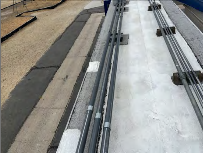
Overview of Roof Area
