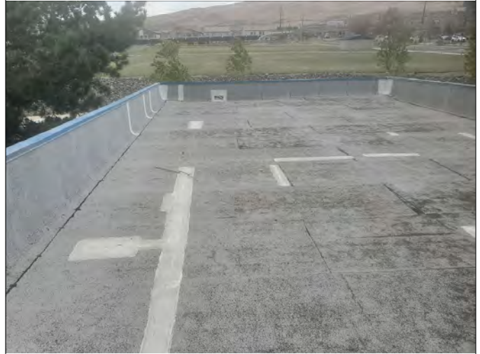
Overview of Roof Area
