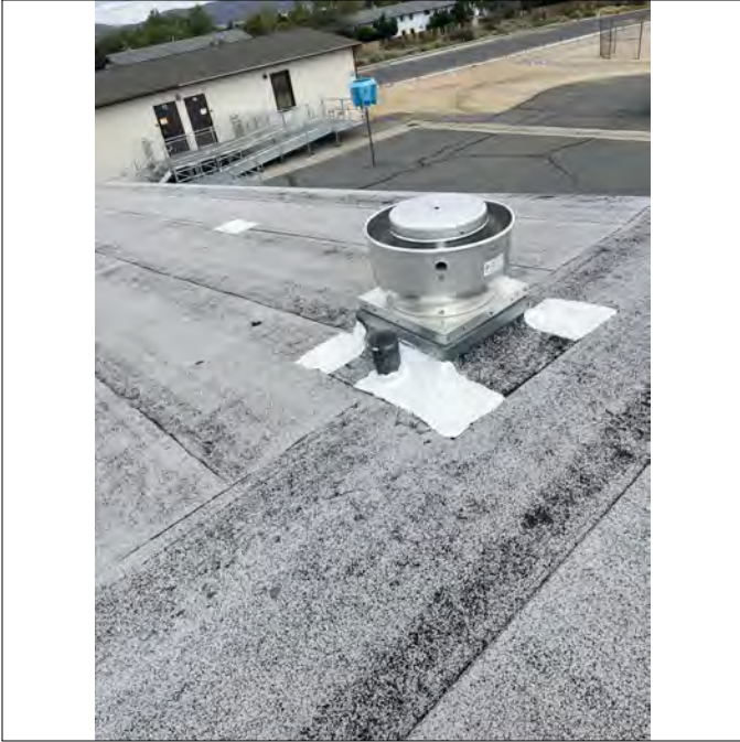
Overview of Roof Area
