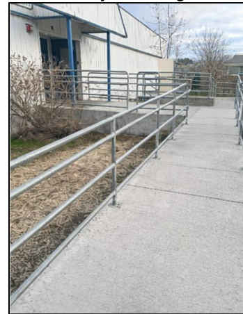
Concrete walk/ramp to Building M
