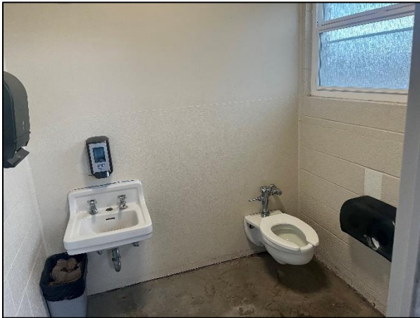
Exterior restroom, Building A (east side of bldg.)
