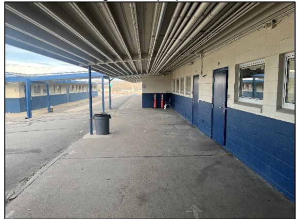
Building B exterior
