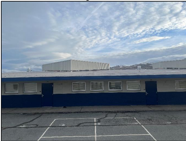
Looking south at Building A exterior/roof system
