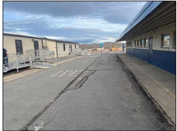
Looking east between Building A and portables
