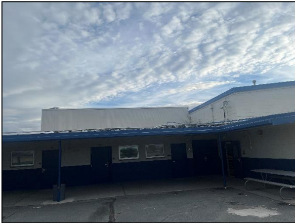
Building B exterior
