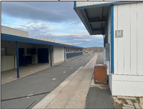
Looking east between Building E & M (near the SWC of site)
