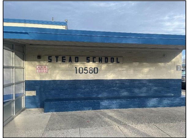
Building B Exterior
