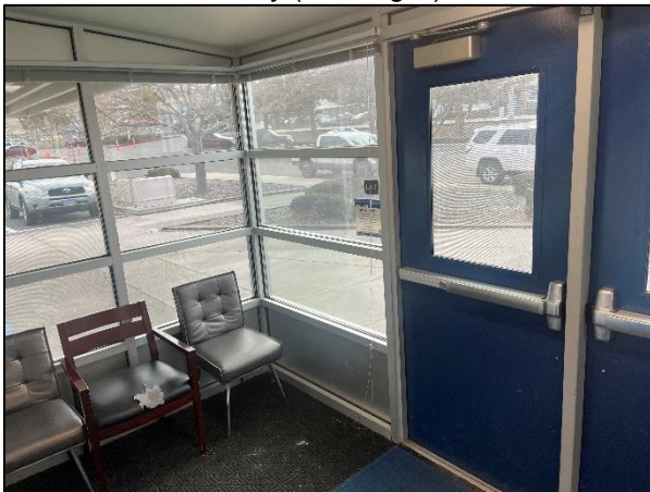
Entry lobby/vestibule (Building B)
