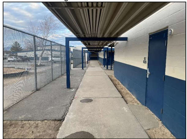
Looking north along front Building E (west side)
