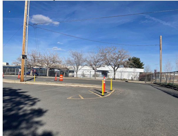
South Side View and Front of Building M, Looking Easterly
