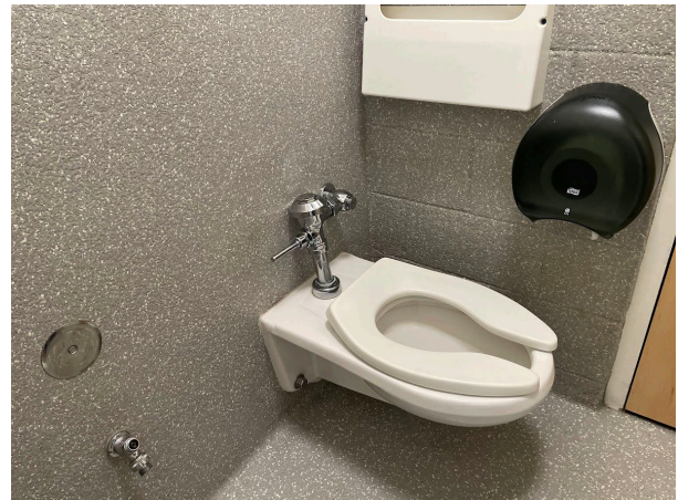
Typical Restroom in Classroom (one per classroom)
