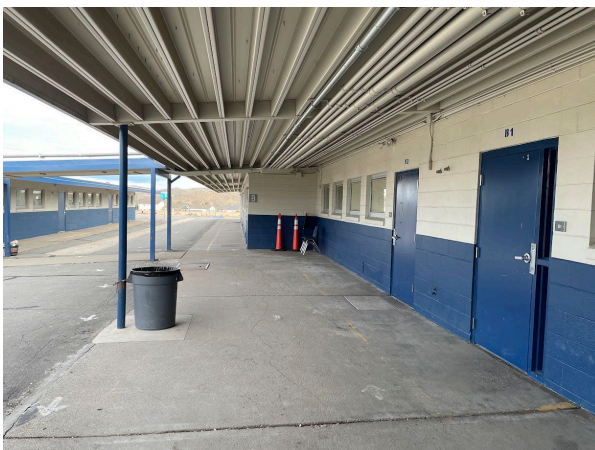
Center/ Main Building Housing Classrooms and Multi-Purpose Room, Looking Easterly
