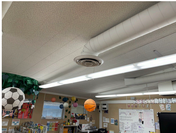
Typical Ceiling Finishes in Classrooms
