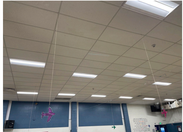
Ceiling Finishes Within Multi-purpose Room
