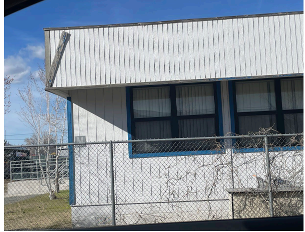
View of Building M, Looking Northerly
