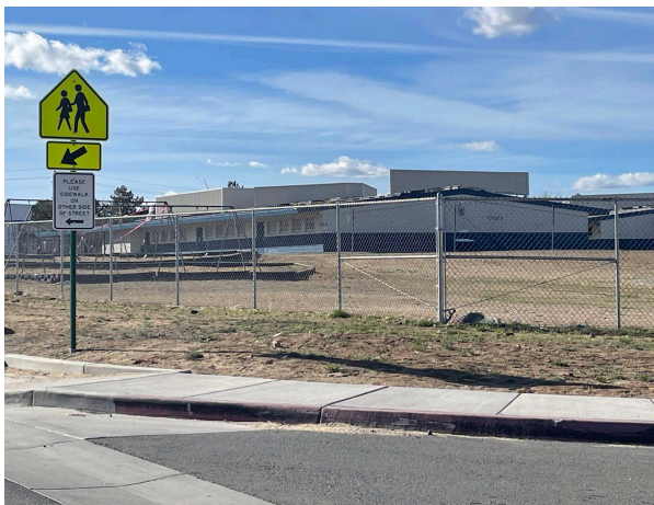
View of School Buildings and Play Area, Looking Northwesterly
