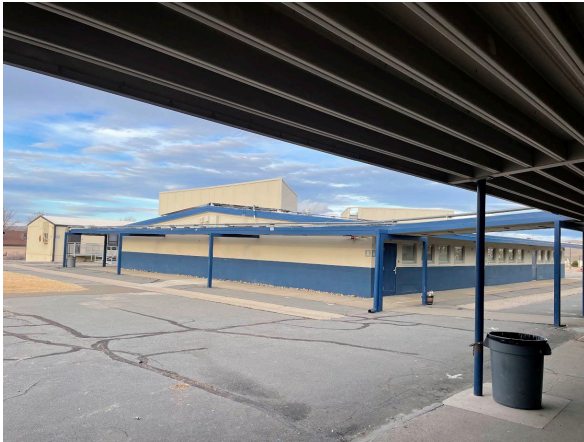
Easterly Building, Looking Northeasterly
