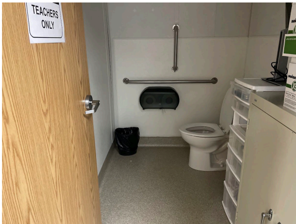
One of Two Restrooms within Mobile
