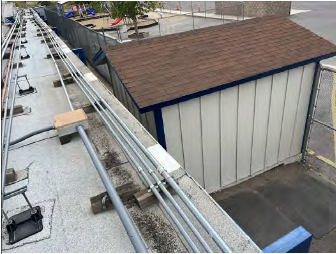
Overview of Roof Area
