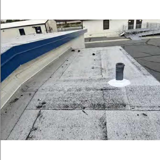
Deteriorated Surfacing
