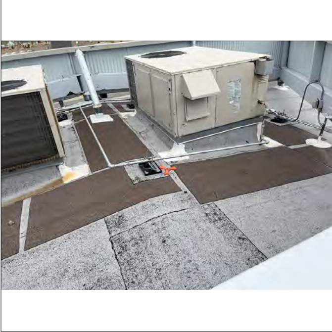
Overview of Roof Area
